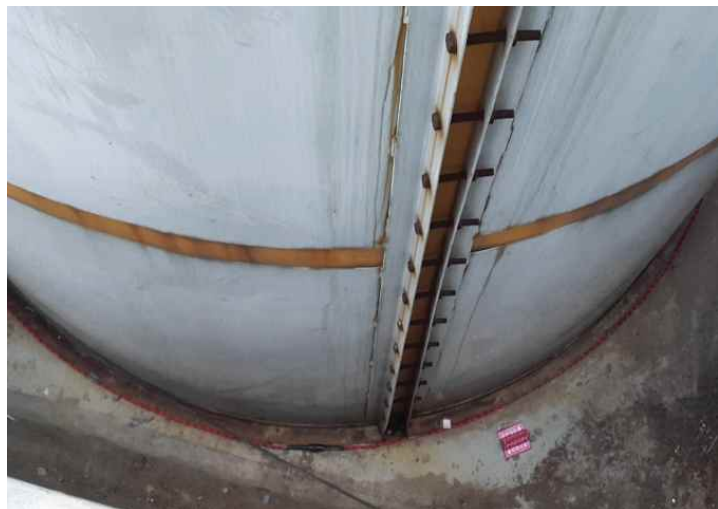
Photo 2. Outdoor Sulphur Hydroxide detection system in Korea Circuit(Ansan)
