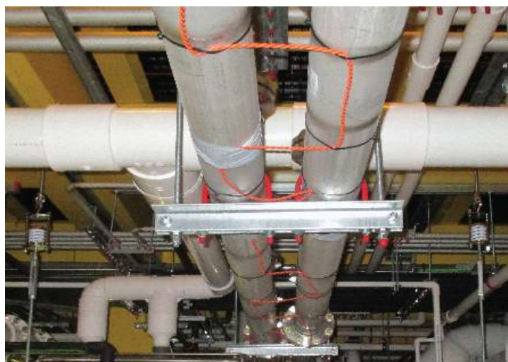
Photo 1. Pipeline leakage monitoring system in LGD(Paju)
